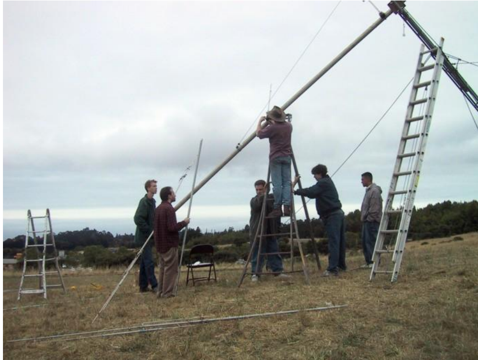
Steve Petersen, AC6P gives instruction as assembly of the HF beam continues.
